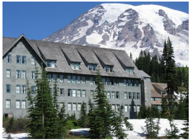
Paradise Inn reflects an alpine variant of the National Park Rustic style of architecture.
